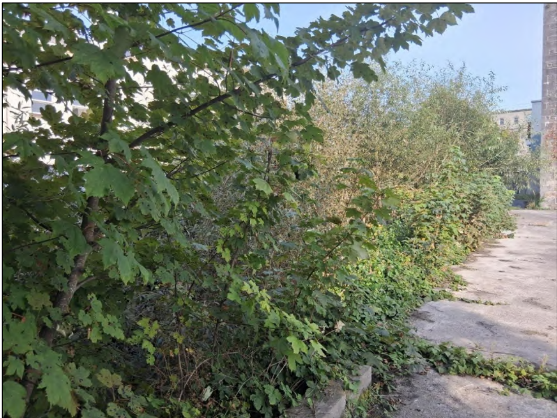
Plate 3-3 Stone wall (BL1) and treeline (WL2) at western edge of concrete yard above the Gaol River to the south of the McLaughlin Building
