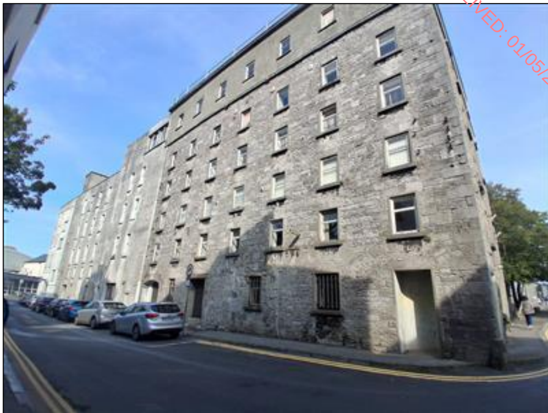
Plate 3-1 McLaughlin Building Southern façade (BL3)
