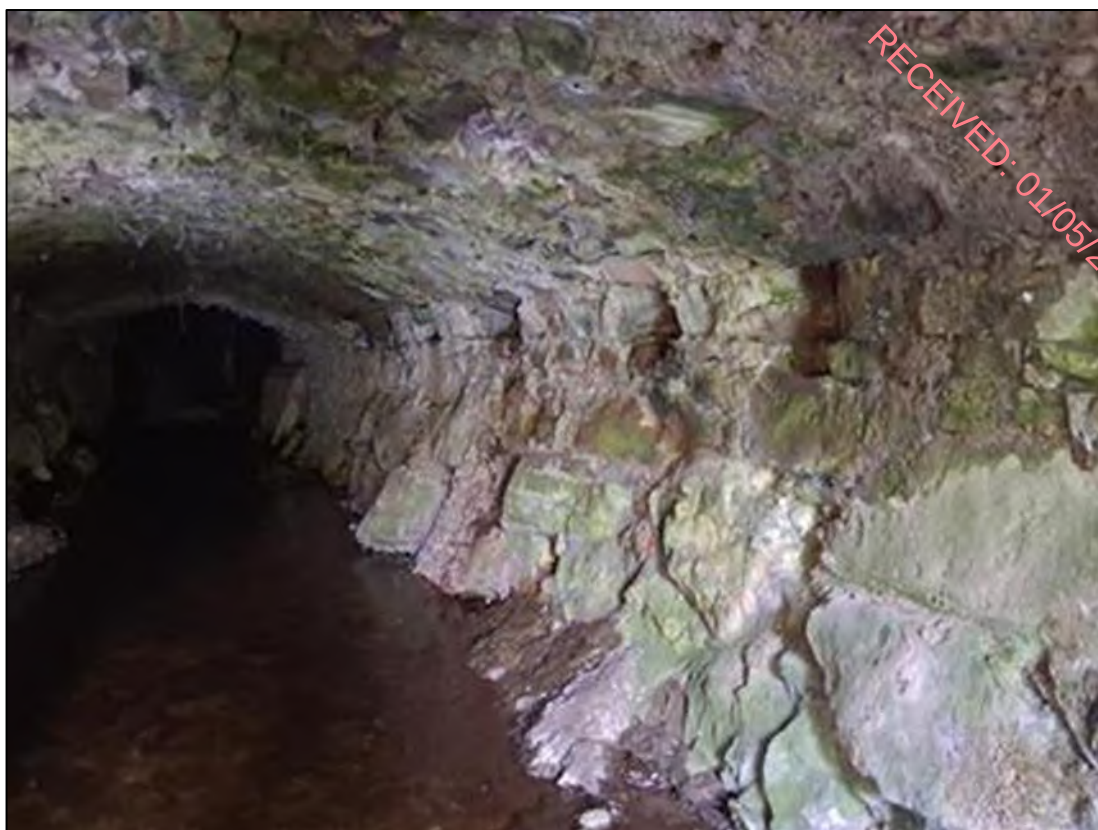
Plate 3-4 Culvert (BL1) under the McLaughlin Building
