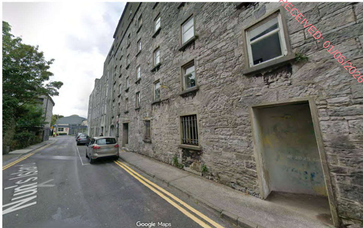
Photo 1.1: Site access off Nun's Island Road to the south of the building
