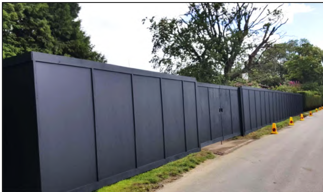
Photo 7.1: Typical Site Hoarding Arrangement
